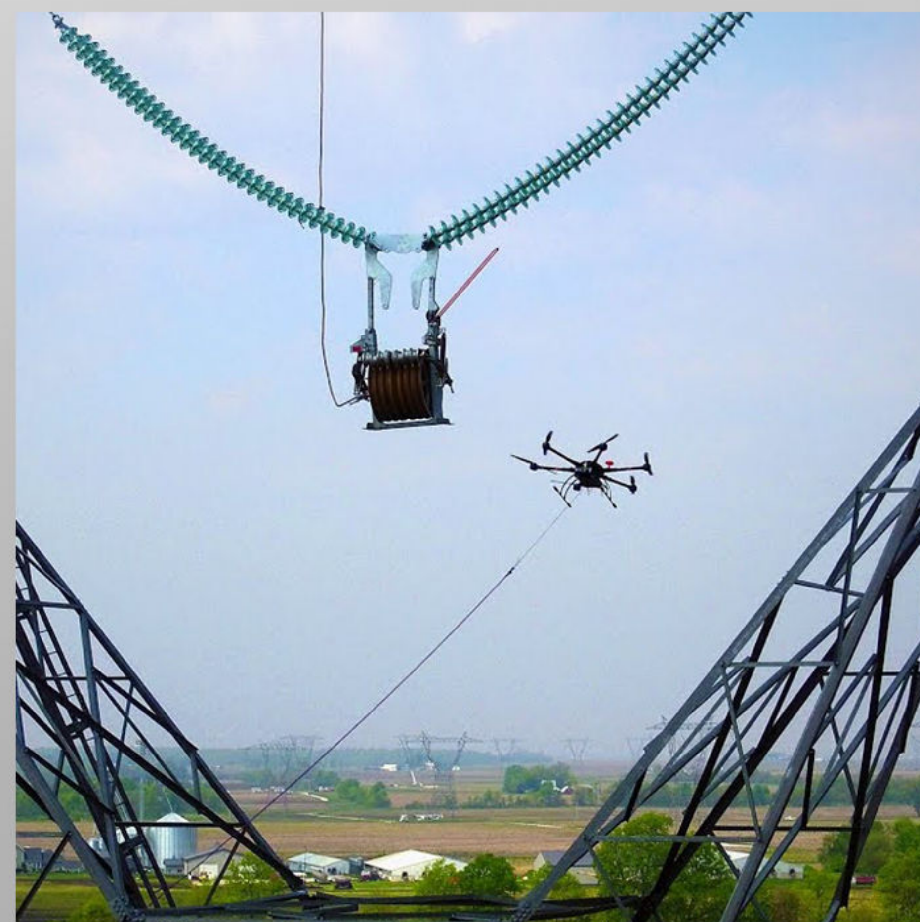
Dron Stringing Transmission Line
