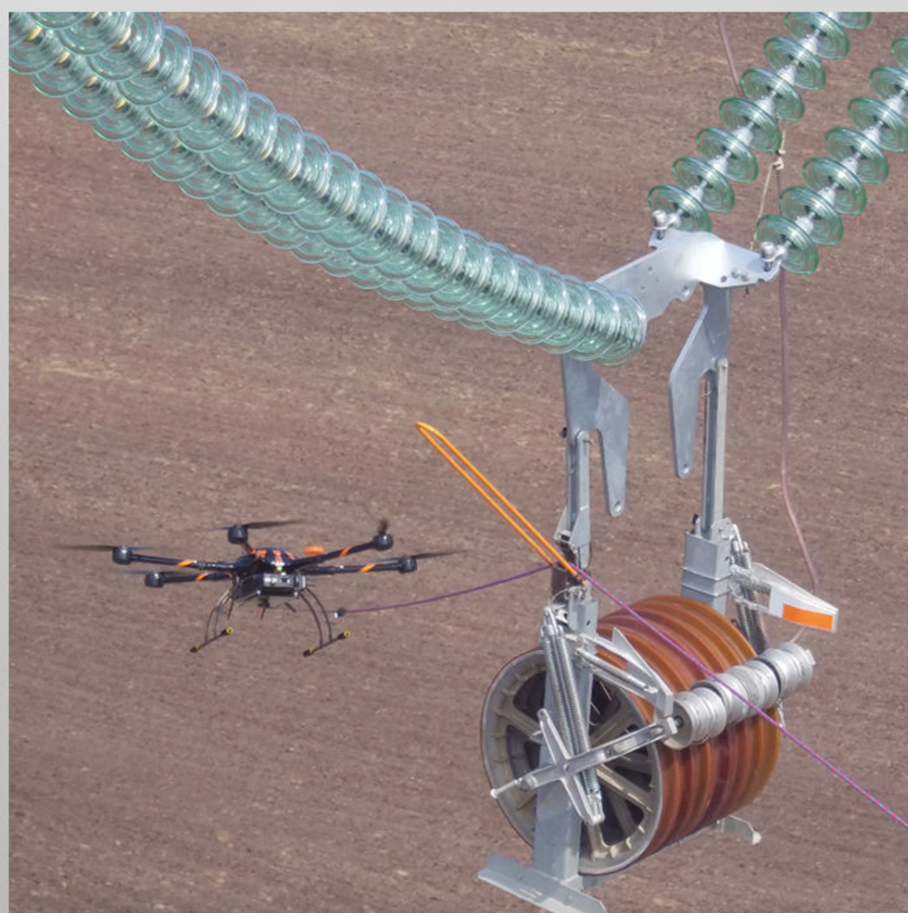
Drones Change Power Line Stringing
